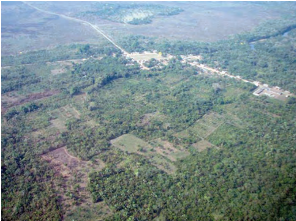
Figure 11.3. The Amazonian settlement and adjacent landscape of gardens, fields, agroforestry, roads, paths, orchards, garbage middens, and forest regrowth at various stages. The dark circular feature in the center is a pre-Columbian ring ditch site. Jasiaquiri, Baures in 2006. (Clark Erickson)
